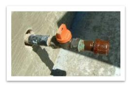
Gas line shut off and capped correctly.
