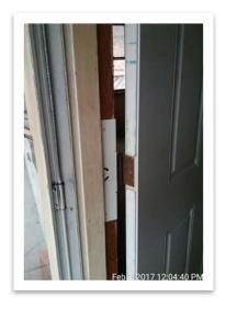
Photo showing door hinge protection product installed.
