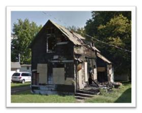
Proper use of boarding and security door on these severely fire damaged properties. The Clear Boarding and Exterior Door Allowables must not be used in these instances.
