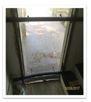
Improper use of clear boarding. Utilize the Exterior Door Allowable to repair/replace missing exterior doors.
