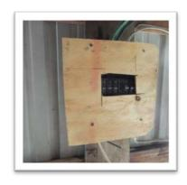
Replace missing exterior electric panels with proper cover. Plywood or clear board is not acceptable.
