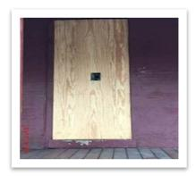
Security door improperly installed leaving no access to the property. Painting of the door to match trim is also required.
