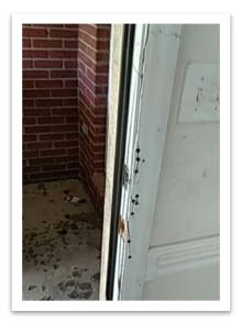
Nailing the door jamb together is not acceptable.
