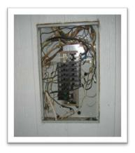
Replace missing exterior electric panels with proper covers.
