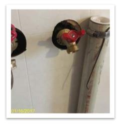
Shut off valve is shown repaired. Capping is now required.
